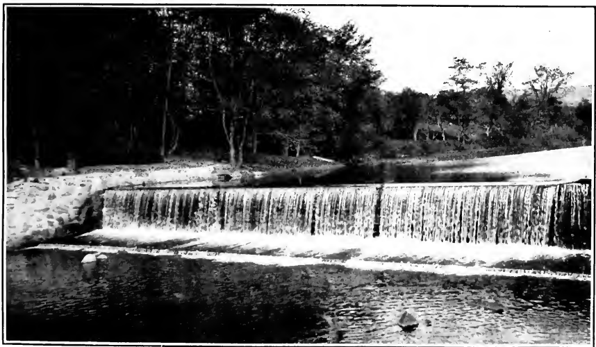
B. DAM ON SWIFT RIVER AT WEST WARE, MASS., OCTOBER 14, 1910.
